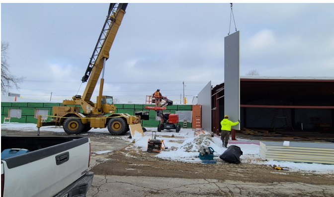
Top row: (L) Construction photos of open office area (R) Showroom/vestibule area Lower row: (L) Installing insulated metal panels on the warehouse addition (R) Warehouse addition
