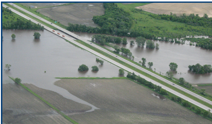
Flooding from the June 2008 storm closed the I-94 westbound roadways for two weeks. Since 2008, the bridges have been placed on a "watchlist" in 2013, 2016, 2018, and 2020.
